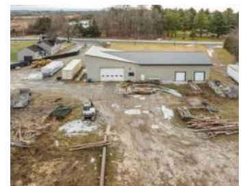
COMMERCIAL - 180,134 PC STANBRIDGE 675 000$ + TX
